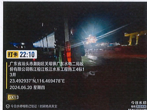
施工4标GX13（南）侧外1米2#
